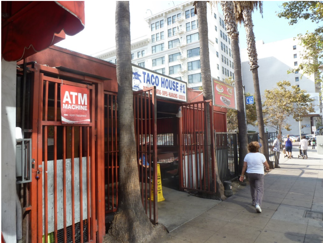
Figure 4: Southeast view of the covered seating area at 348 South Hill Street. Source: GPA
